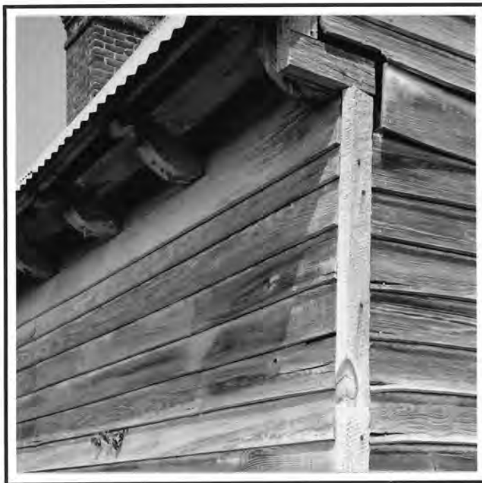
Figure 24. Pear Valley, decorative joist ends carrying tilted false plate. (Photo credit: Willie Graham, Colonial Williamsburg Foundation.)
