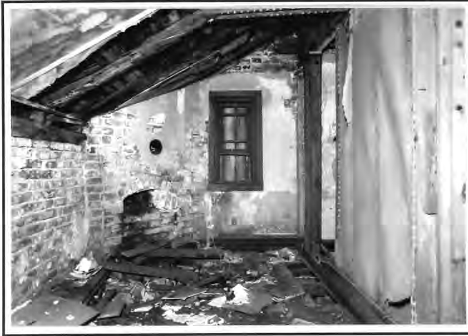
Figure 36. Matthew Jones House, corner fireplace in shed.
