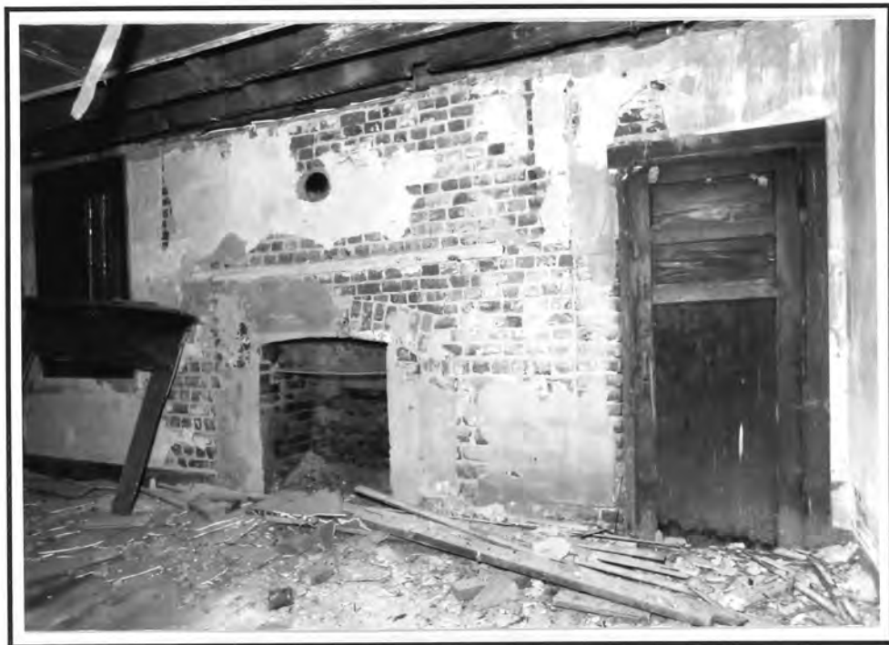
Figure 29. Matthew Jones House, chamber fireplace. New cheeks were added to both sides of the firebox probably in the late nineteenth century.
