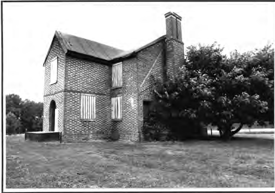
Figure 2. Matthew Jones House, exterior, looking north.
