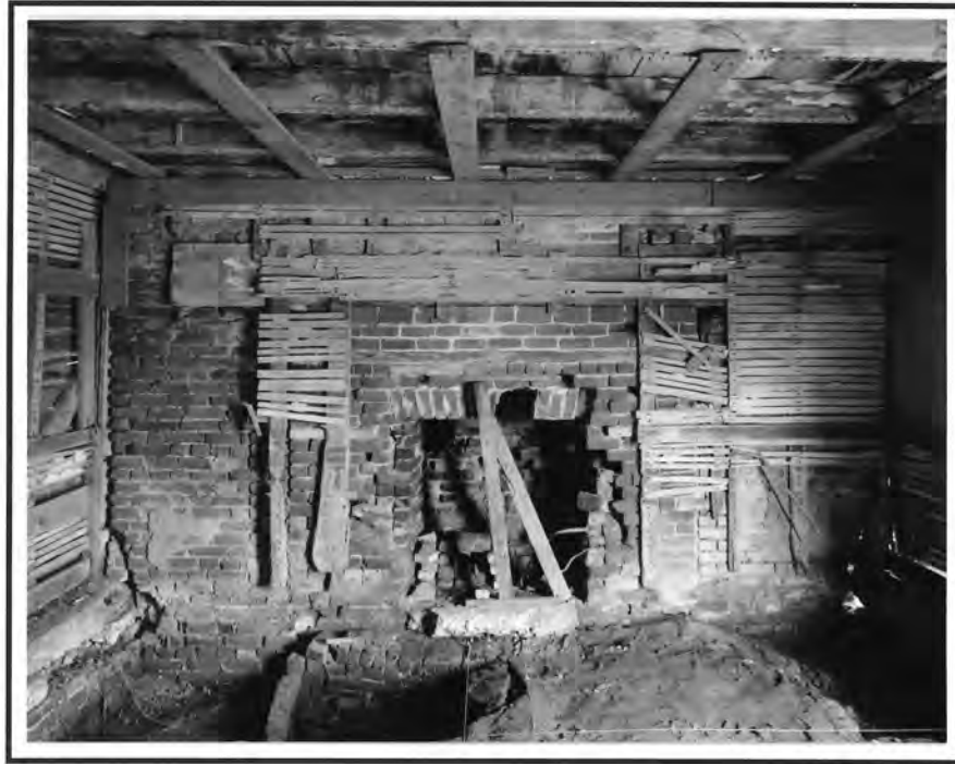
Figure 33. Pear Valley, hall fireplace, originally with an opening nearly 8 ft. wide, was dramatically reduced in size later in the eighteenth century. This example parallels the reduction in scale of the Matthew Jones hall fireplace. (Photo credit: Willie Graham, Colonial Williamsburg Foundation.)
