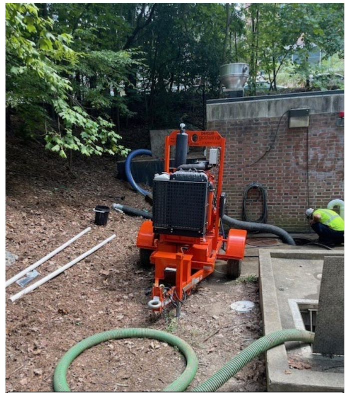
Temporary bypass pump in place to assist the lift station until repairs are completed. Photo taken on 8/27/24
