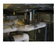
Of the existing equipment, the two newer Trinkle Hall chilled water pumps and the one newer chilled water pump in the Campus Center Building are in good shape and seem to be installed to allow access for servicing.
