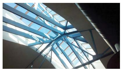
Photograph 2 – Roof framing in the central atrium of Trinkle Hall. In this photograph the primary roof supporting element is a steel truss, while the secondary framing consists of wood joists.
