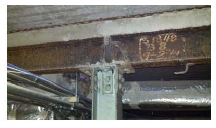
Photograph 3 Photograph 3 illustrates the corroded condition of the structural steel that supports the floor system in the central portion of the building.
