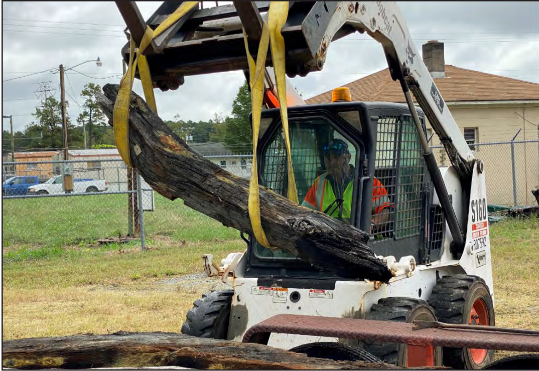
Figure 6.6. VDOT personnel loading floors for transport to TAR facility.
