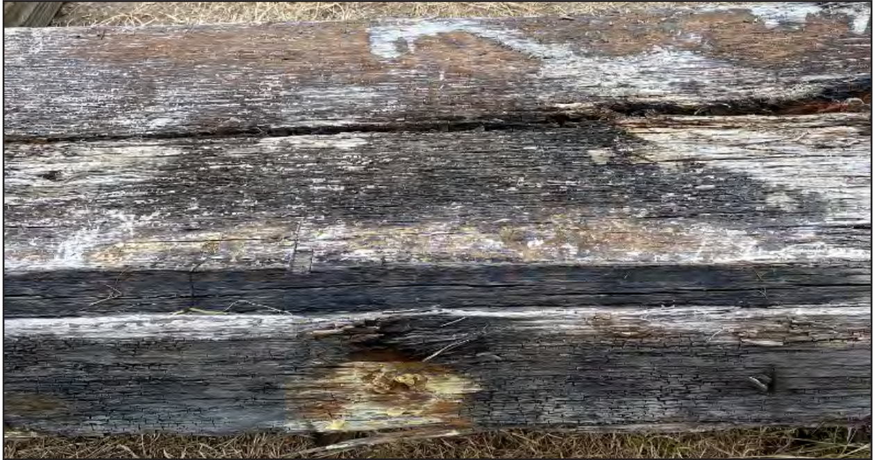
Figure 6.19. Shallow rabbet in top of K-1 section.
