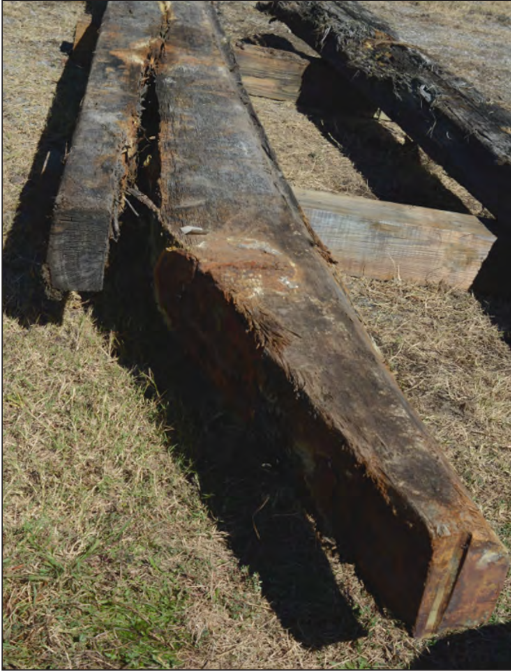
Figure 6.16. Keel scarf looking aft.
