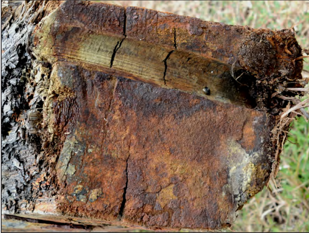
Figure 6.17. Stopwater recess in the forward end of the keel scarf.
