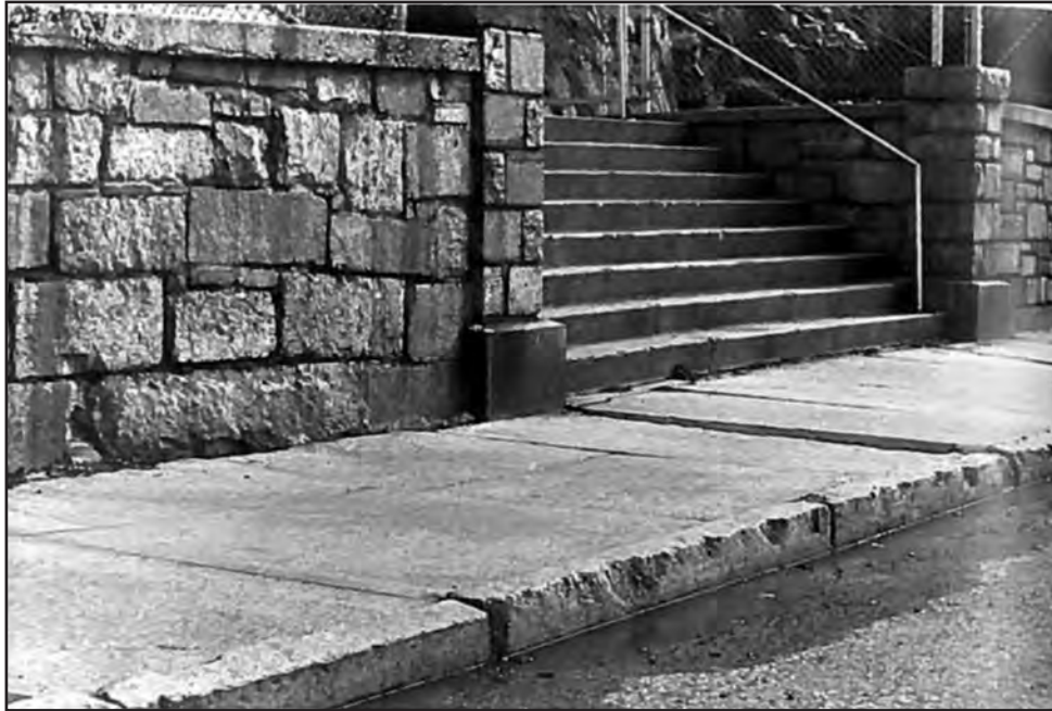
Figure 3.23. Gneiss from Port Deposit quarry used in local construction in Maryland (Blumgart 1996:72).
