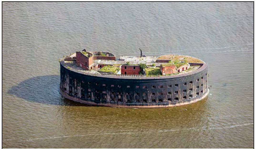
Figure 3.20. Example of a completed fort with three rows of casemates and positions for guns en barbette (Fort Alexander I on the Gulf of Finland near Kronstadt Naval Base and St. Petersburg, Russia [Shiva 2016]).
