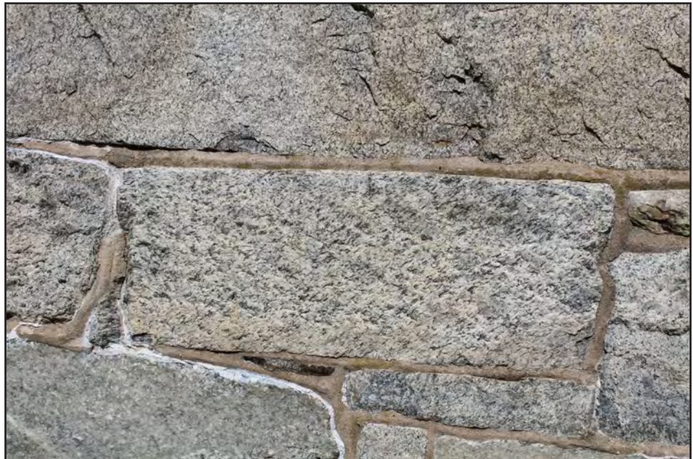
Figure 2.2. Detail of masonry in the Flagstaff Bastion of Fort Monroe.
