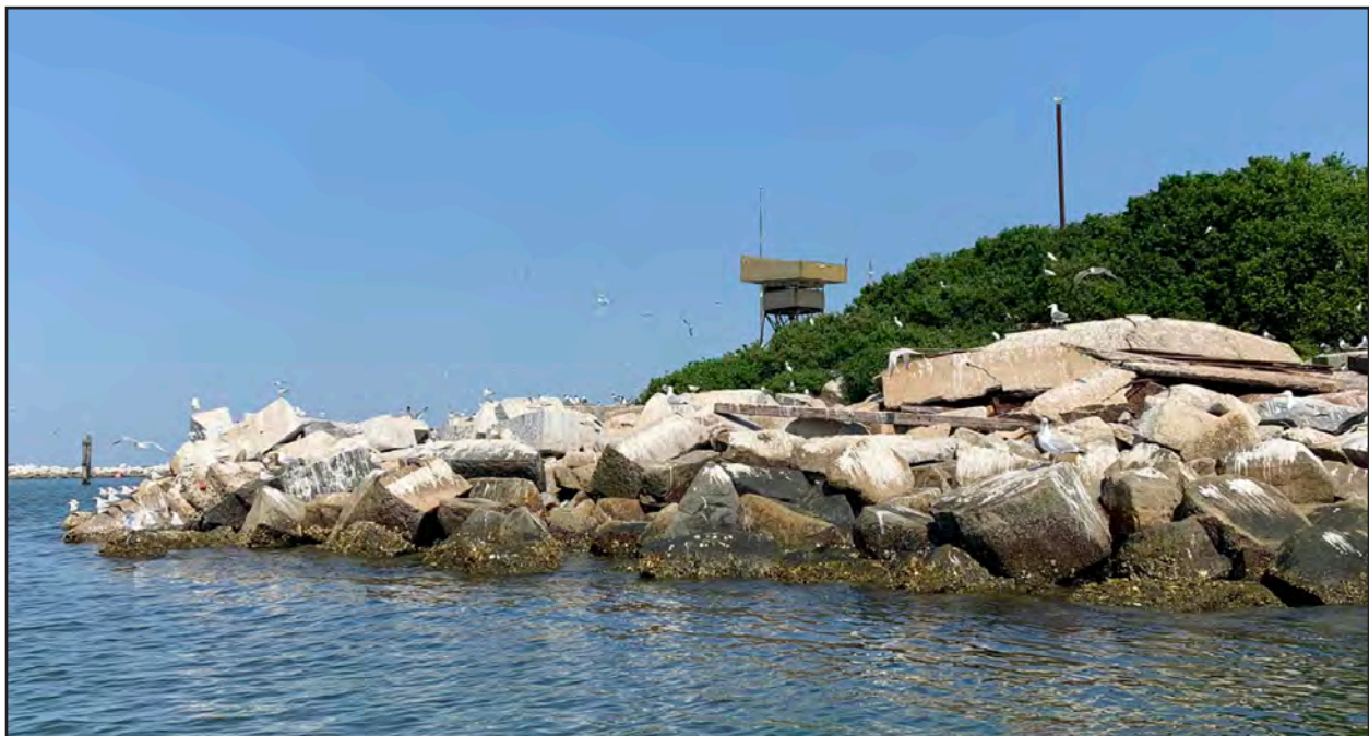
Figure 2.4. Stone block forming southeast portion of artificial island built up from underlying Willoughby Shoal for the construction of Fort Calhoun/Fort Wool.
