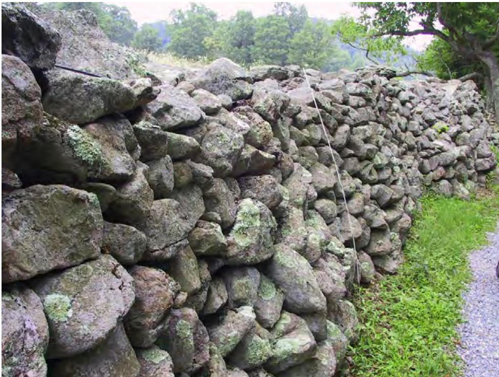
Figure 22. View along the face of the west wall at the lower end of lane, looking north. (Measuring stick is 6.6 ft.)
