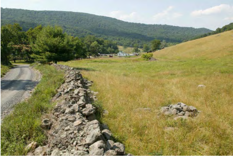
Figure 47. Roadside wall, looking west toward Giles Partlow farmhouse.
