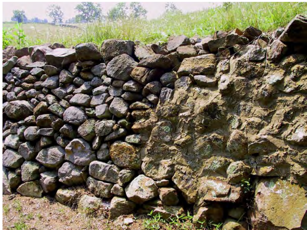
Figure 66. Retaining wall just south of Running Brook farmhouse. Originally drylaid, a portion (right) has been reinforced with mortar.
