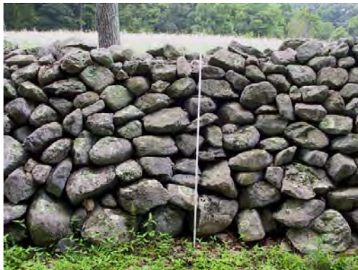
Figure 21. Elevation view of high west wall at the lower end of lane. (Measuring stick is 6.6 ft.)
