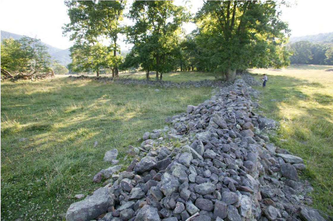
Figure 60. View of collapsed main wall, looking west from Area 11.
