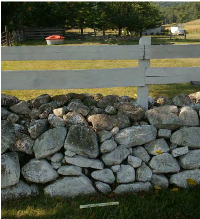
Figure 52. Detail of wall on north side of driveway topped with wooden fence.
