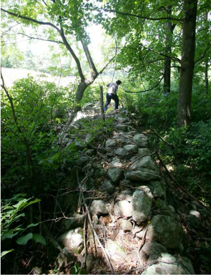
Figure 29. Top of massive wall that parallels upper portion of Gooney Run, looking north.
