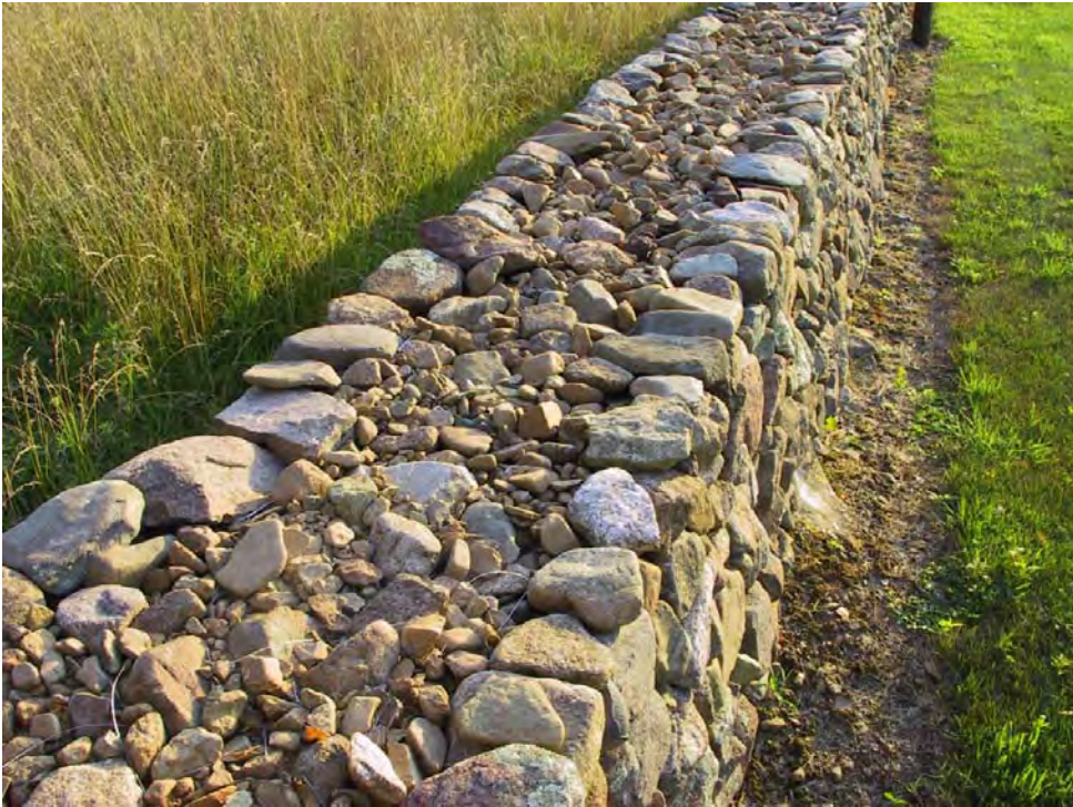
Figure 71. Top of wall rebuilt by Clem brothers showing rubble infill.
