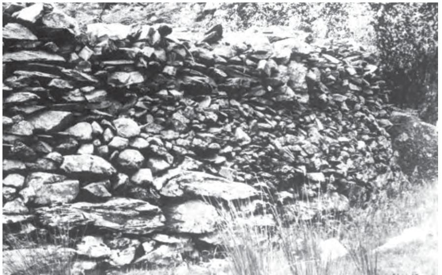
Figure 74. Although more straight-sided than the walls at Gooney Manor, this Welsh "consumption" wall represents similar purpose and informal construction. Garner (1997:8) notes the wall's bulk compensates for its haphazard arrangement of stone, preventing the wall from collapsing.
