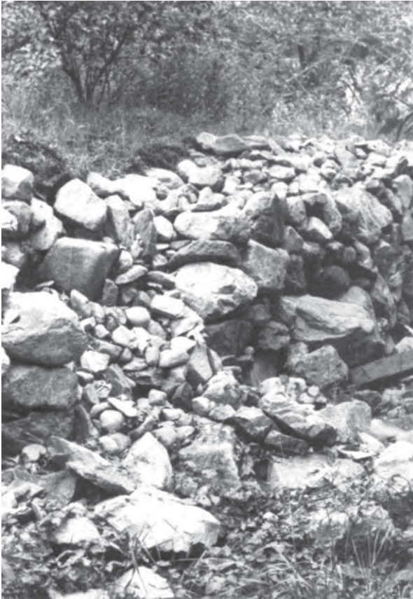
Figure 75. Partially collapsed New England walls made of smoothed glacial rock (Wooley and Raitz 1992:100).
