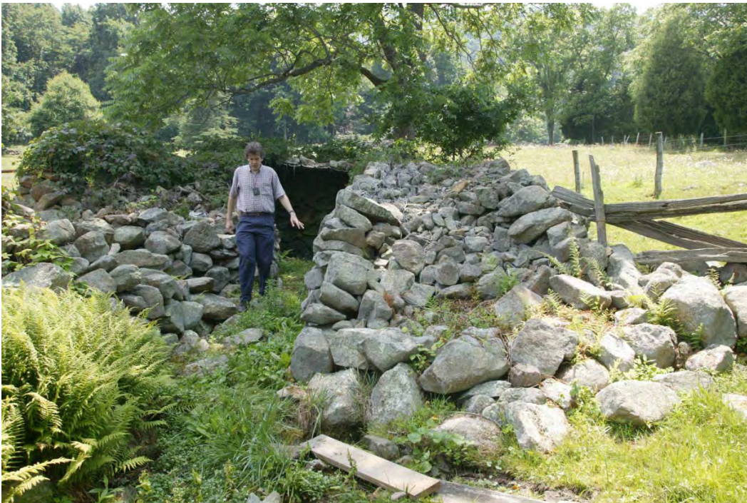
Figure 36. Spring enclosure and mound, looking south.
