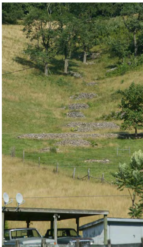
Figure 54. Check dams in gully, looking southeast.
