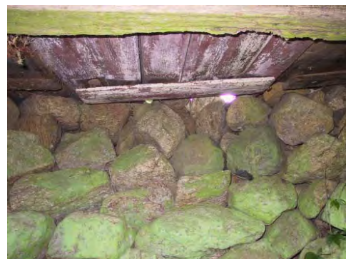
Figure 41. Roof of spring chamber.
