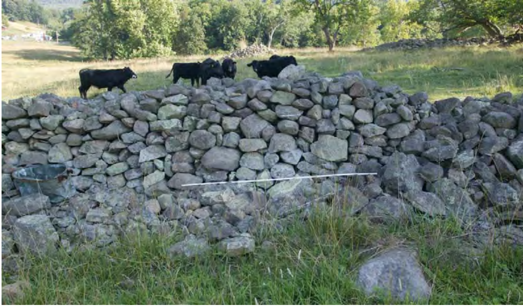
Figure 59. Elevation at Area 11, looking south.
