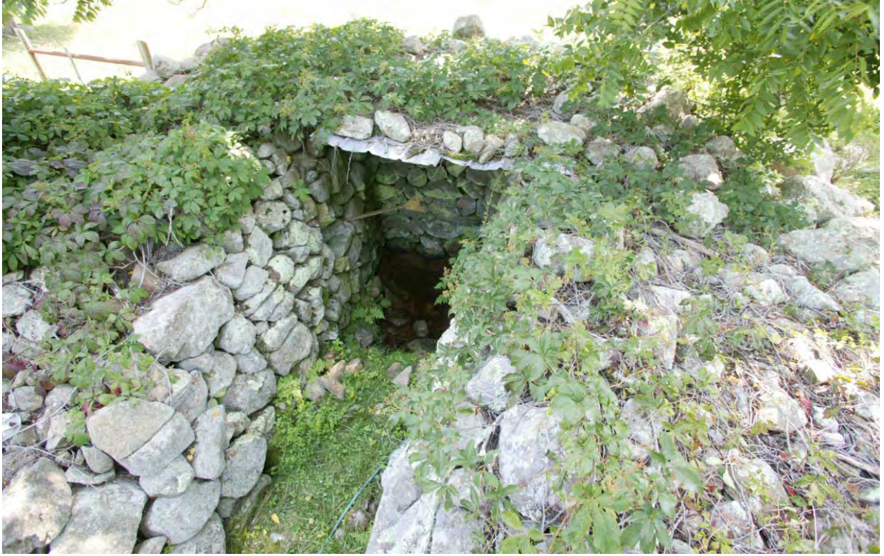
Figure 37. Overhead view of entranceway to spring enclosure.
