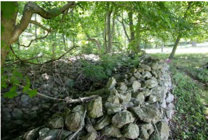
Figure 30. Twin walls alongside upper portion of Gooney Run, looking south.
