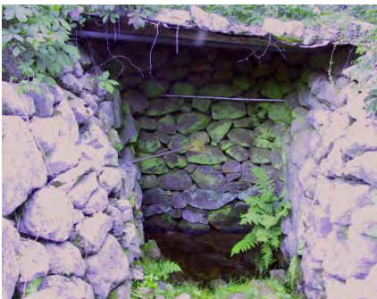
Figure 40. Detail of spring chamber.
