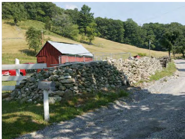
Figure 49. Roadside wall on south side of driveway, looking southeast.
