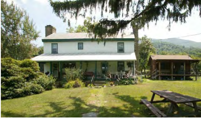
Figure 34. Perna farmhouse and front yard, looking south.
