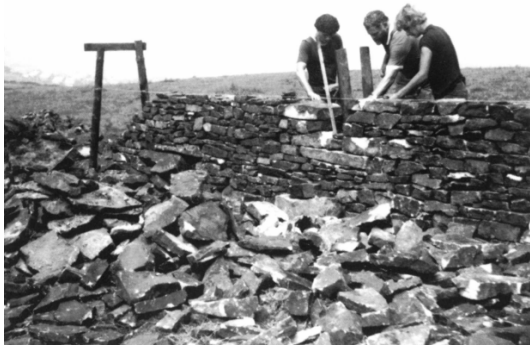
Figure 24. The wooden template at left shows the steep sides and height of wall necessary for enclosing sheep. Note the dressed stone used in such a finished enclosure wall (Garner 1997:13).
