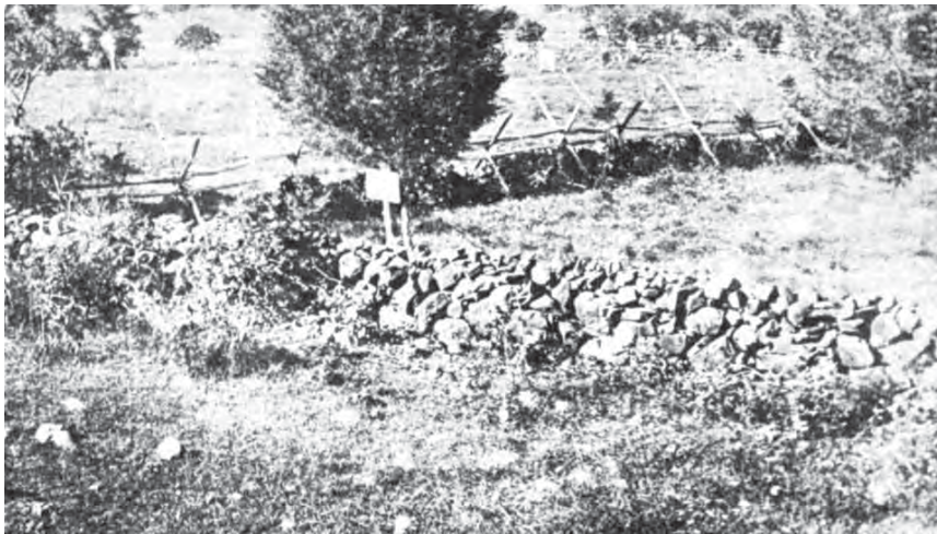
Figure 76. Stone walls in front of Giles Partlow farmhouse (above) and on the battlefield at Gettysburg, Pennsylvania (left, Horan 1955:Plate 138), both supplemented by wood fencing. With these adaptations, a low wall becomes an effective enclosure while considerably reducing expenditure on timber. Also, posts supported by cobbles (above) would resist rot much longer than when planted in the moist ground.
