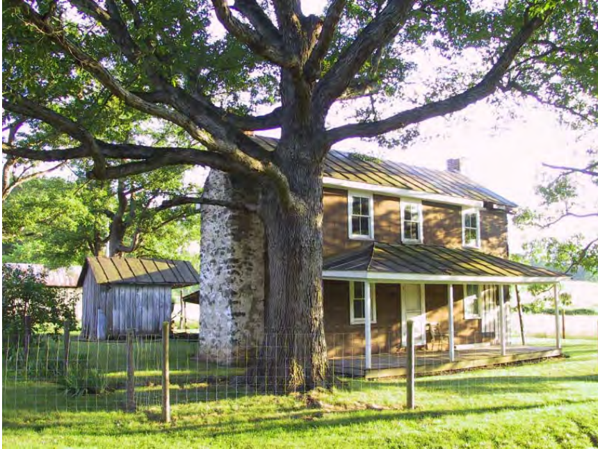
Figure 69. Thornhill (94-205), looking southwest.
