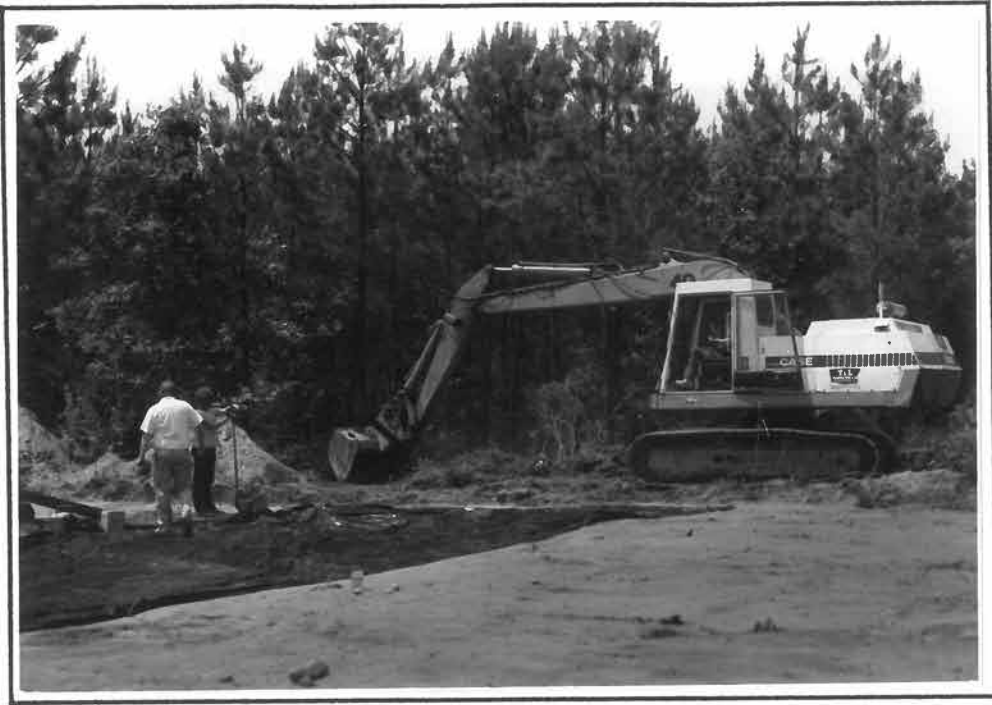
FIGURE 7 Mechanical removal of vegetation and plowzone overburden at Site 44CC297.
